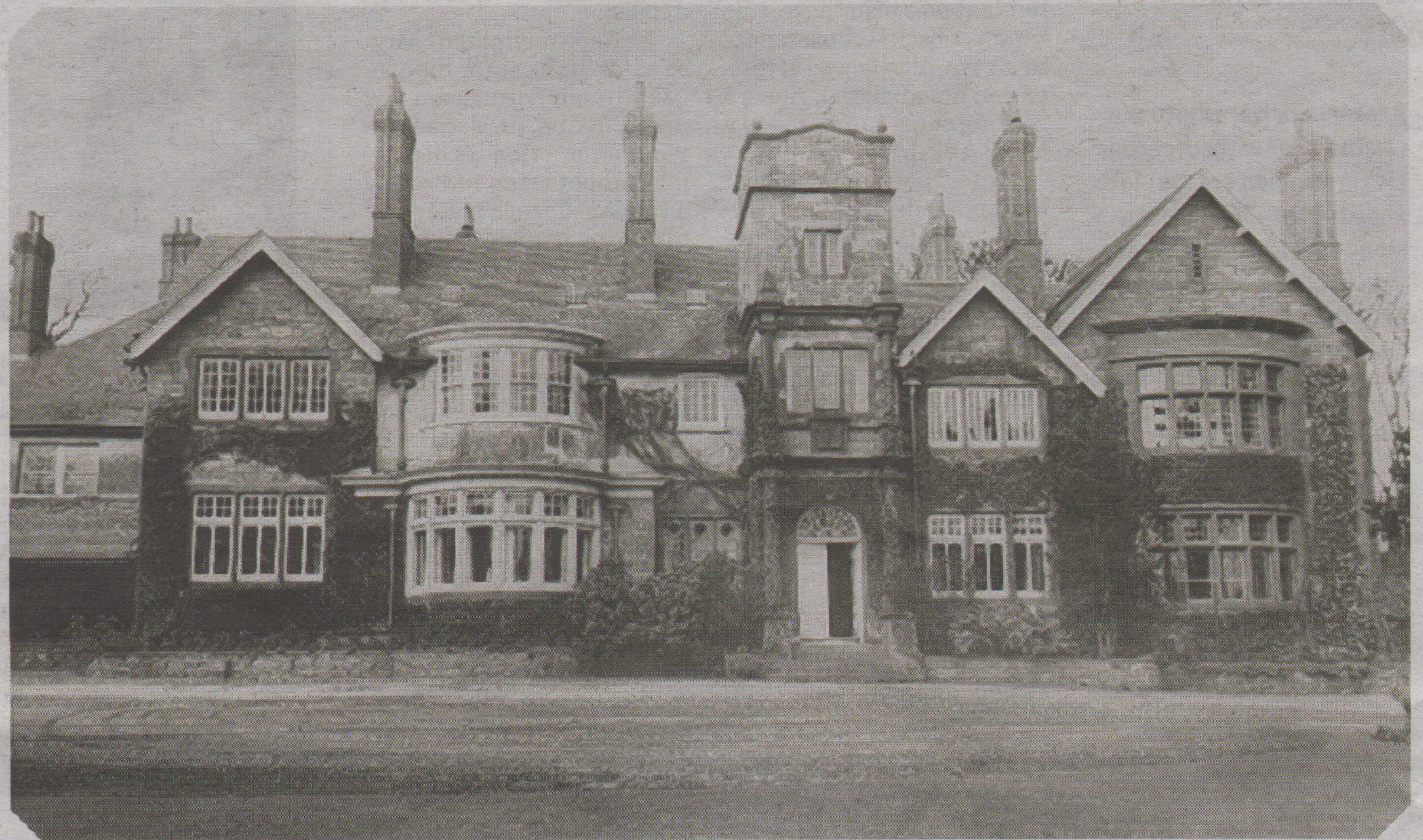
Billown Mansion, Malew, Rigby's largest commission, designed for the Moore family. In addition to the mansion house his brief included a model farm, lodges, motor garage and estate houses. The mansion replaced an older house called Crescent Cottage. The scheme was so great by local standards that two Castletown builders had to combine forces to complete it, Coopers and Corrins
